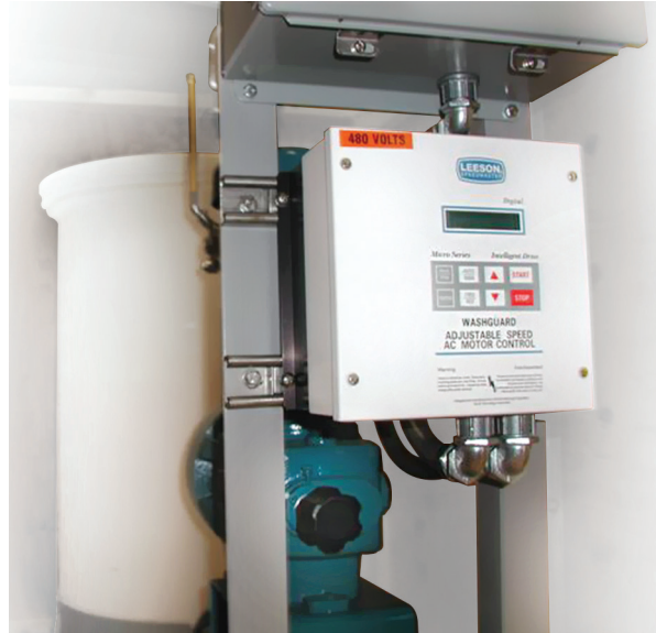
Variable Speed Driven Chemical Dosing System
